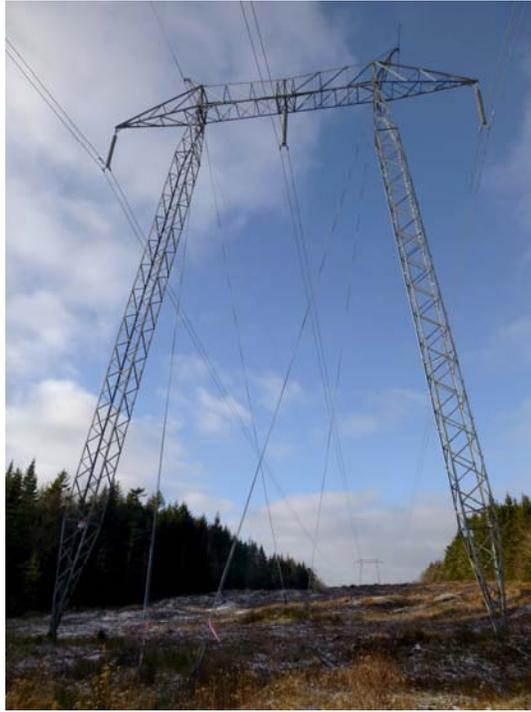
**Figure 1: Sample photos of guyed transmission towers**
